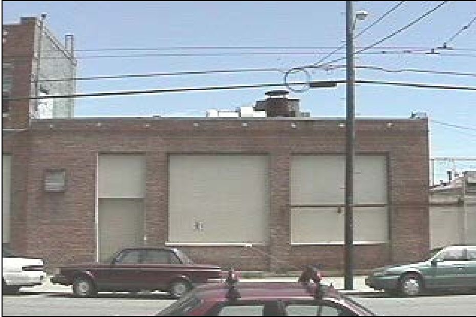
Photo 2. View of single-story section from Tennessee Street looking east. May 14, 2001.
