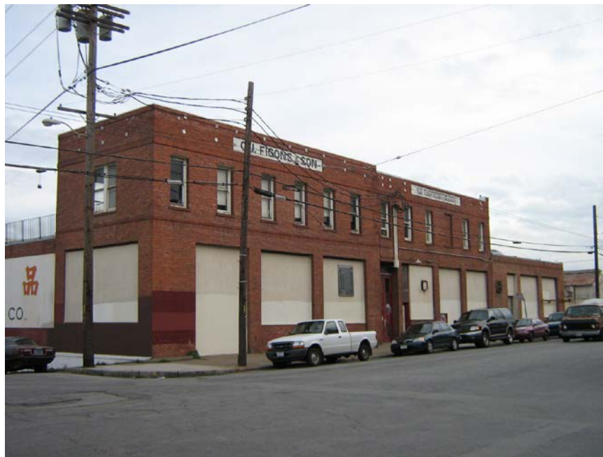
815-825 Tennessee Street, primary façade (6 February 2007)
