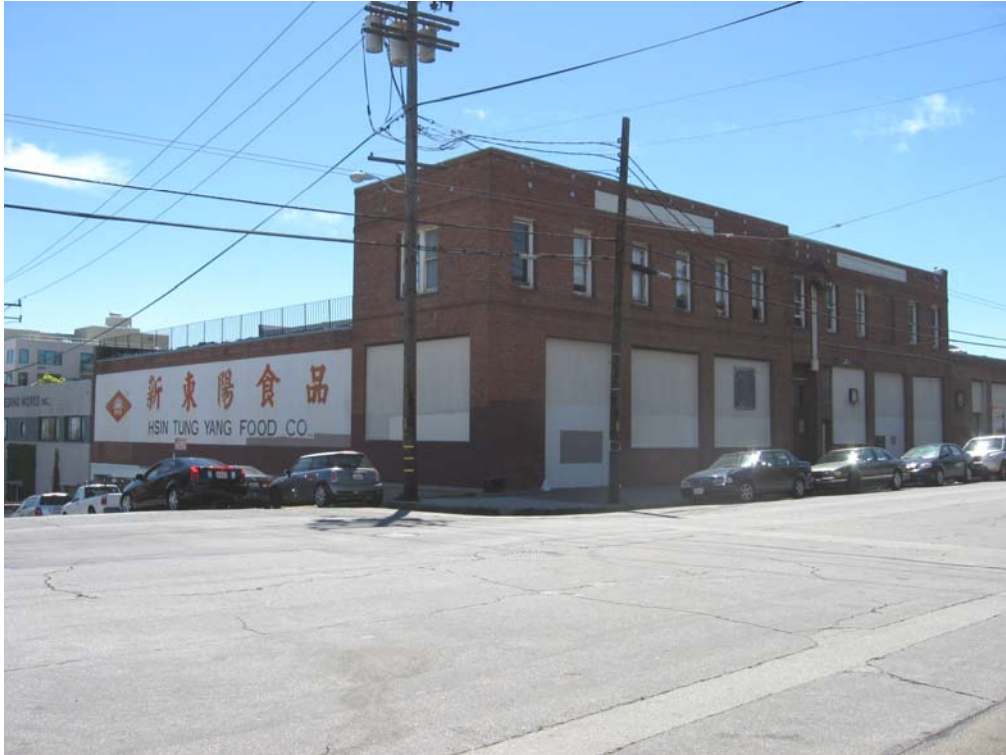
North and primary (west) façades, looking southeast.
