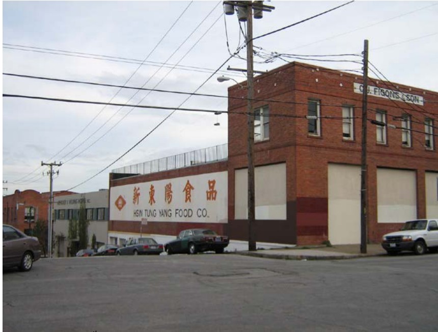
Corner of 19 th & Tennessee Streets, looking southeast (6 February 2007)
