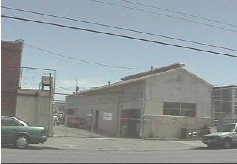
Photo 4. View from Tennessee Street looking southeast. May 14, 2001.
