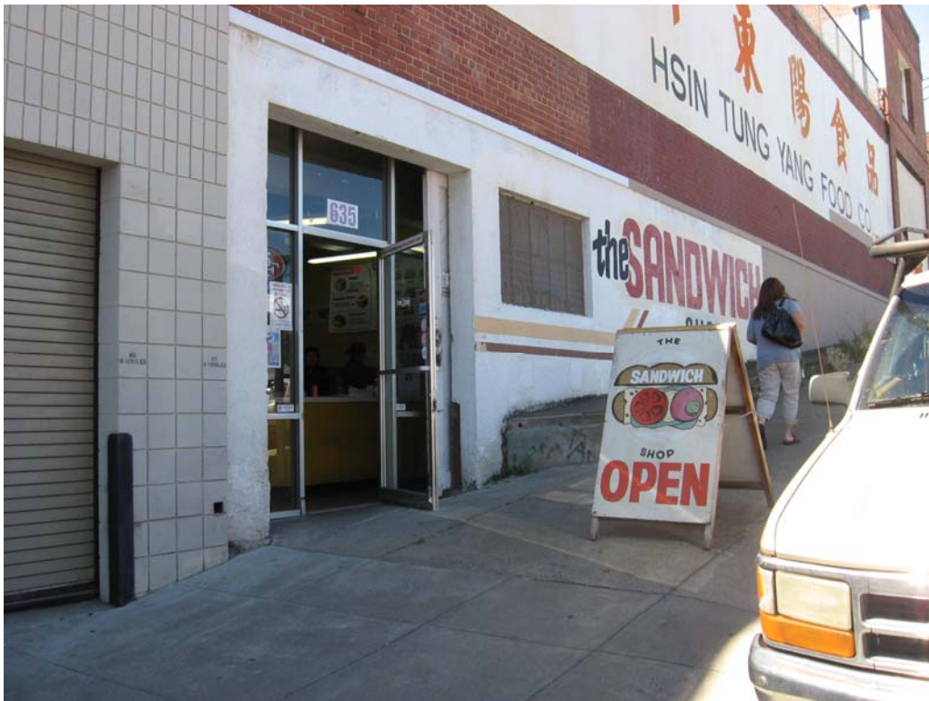
Detail of basement entrance at east end of north façade.
