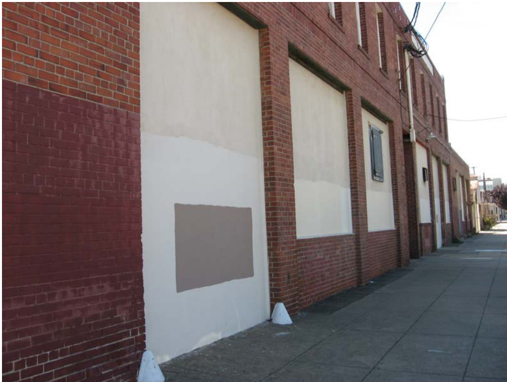
Detail of infilled openings on primary (west) façade, looking south.
