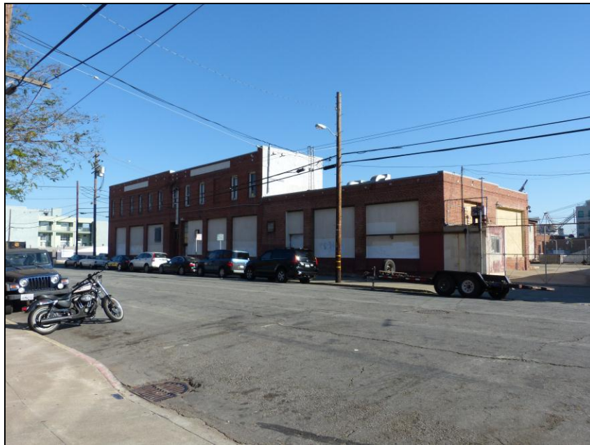
Photograph 1: 815-825 Tennessee Street, primary (west) façade Photograph taken by Tetra Tech November 1, 2013
