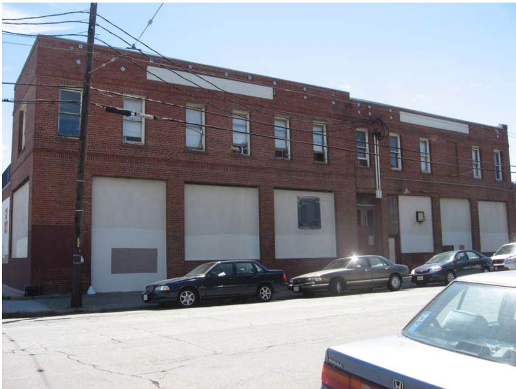
Primary (west) façade, looking southeast.
