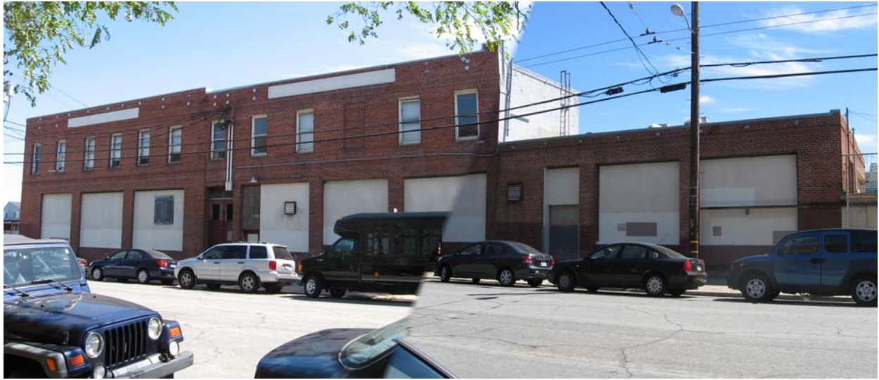
Primary (west) façade, looking east.
