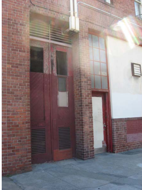
Detail of two entrances at center of primary (west) facade.
