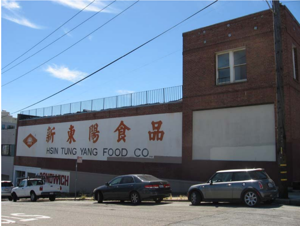
North façade, looking southeast.
